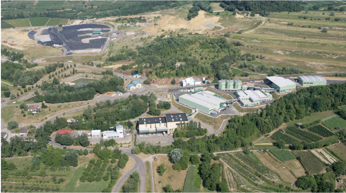
Kahlenberg (ZAK) MBT plant, Ringsheim [6]
